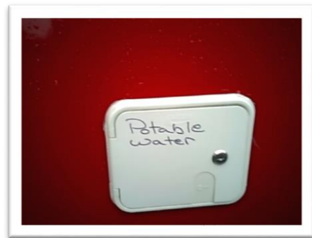
Potable Water Inlet
