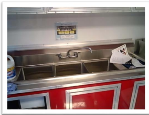
Three-compartment sink
